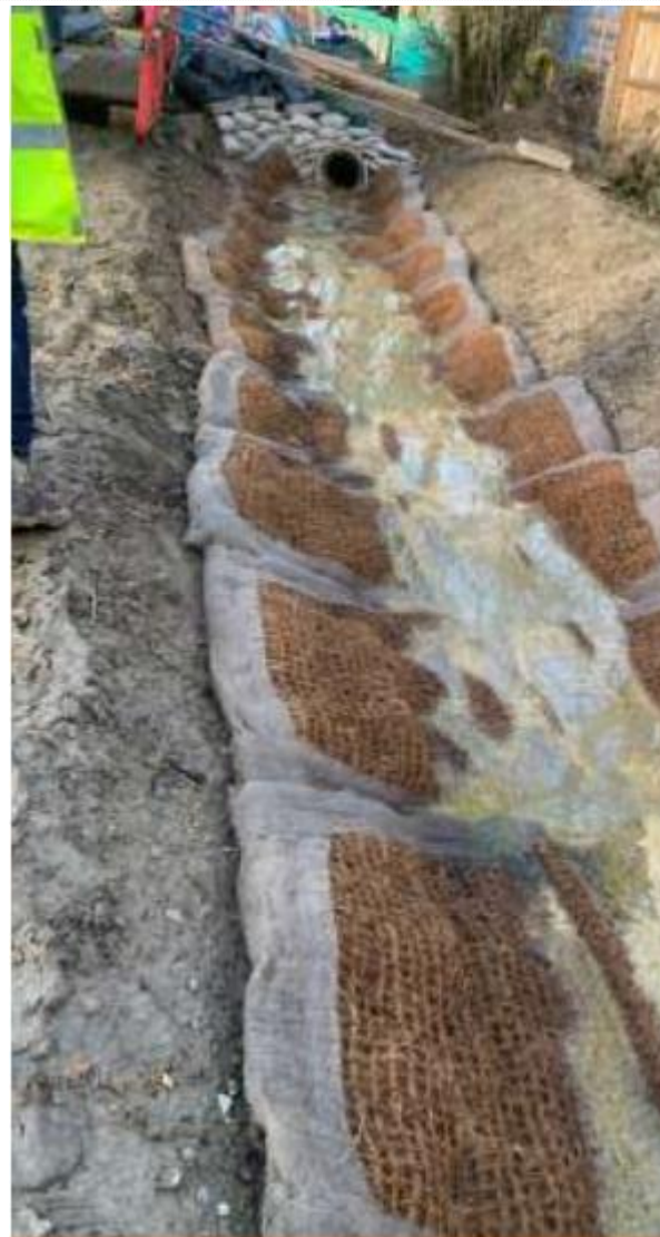
Trench with flocculant matting
